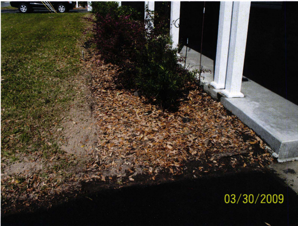
Picture 1: 269 Birch Drive UST excavation site.
