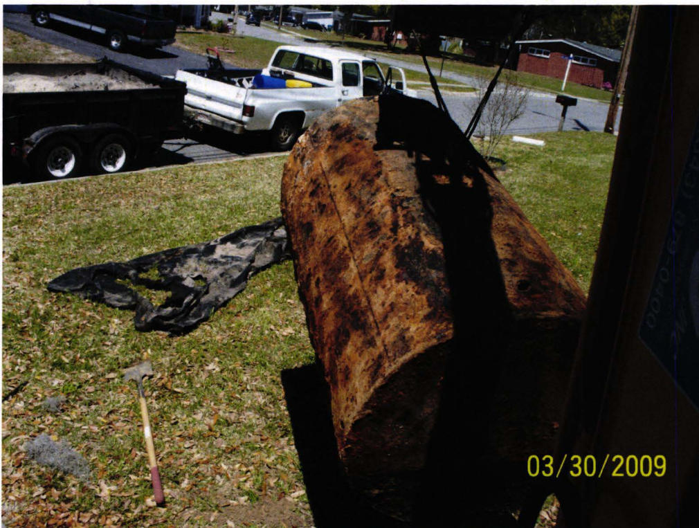
Picture 2: UST 269Birch after removal from the excavation.
